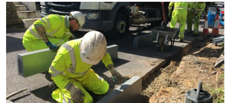
Laying recycled plastic kerbs in Hampshire
